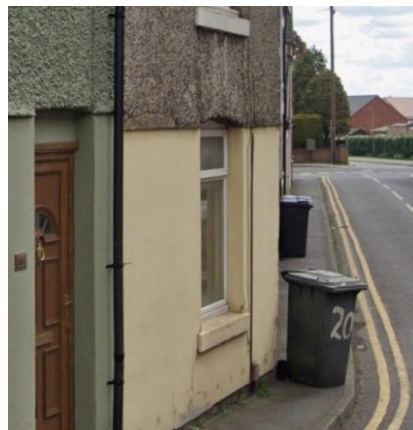
Image 16: Narrow pavement between 14 and 22 Breach Road, Coalville
