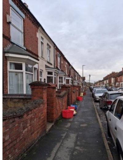
Image 9: Terraced dwellings with frontage. Park Road, Coalville.
