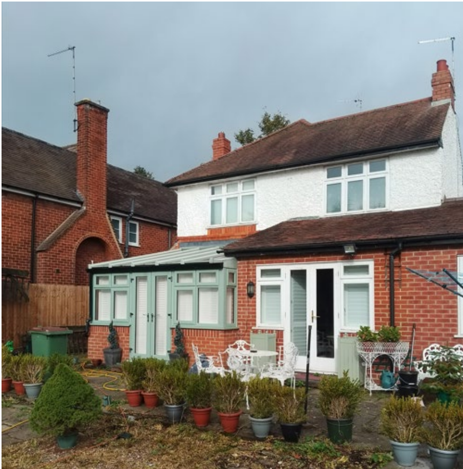
Rear elevation adjacent to Ringwood
