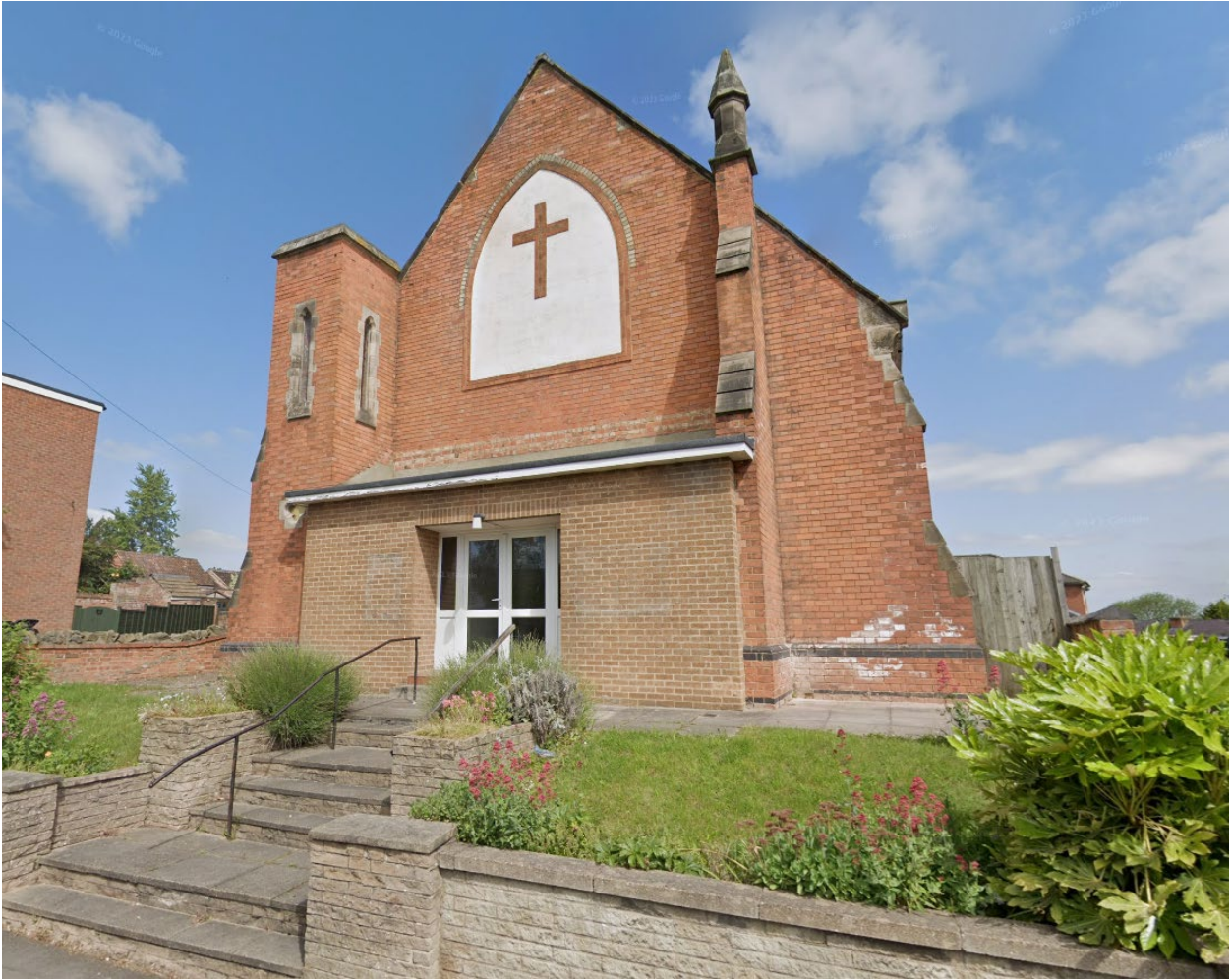
View looking directly to the frontage of the church
