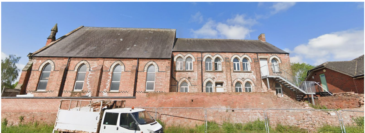
View of the publicly visible east elevation of the church
