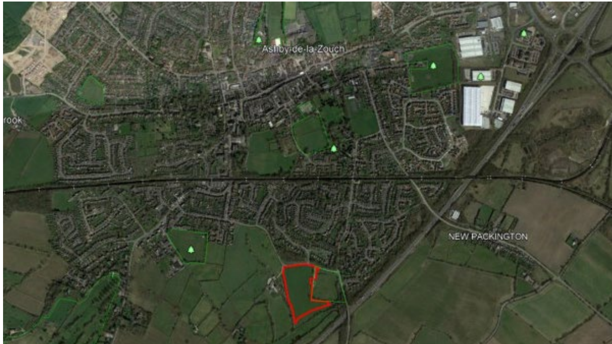
Aerial view of the site
