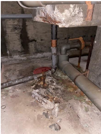
Corrosion of Reinforcement Within Structural Concrete
