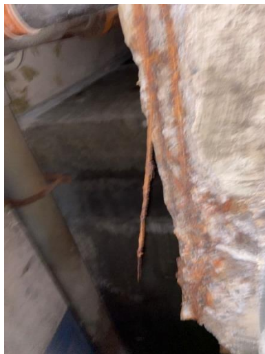
Corrosion of Reinforcement Within Structural Concrete
