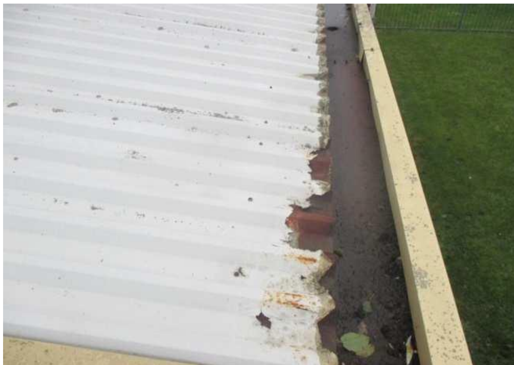
Corroded Edges to Cladding
