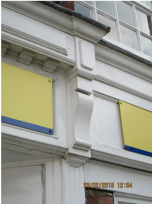
34A Market Street, Ashby. c.1930. A fluted pilaster carries a simple scroll bracket. The cornice is advanced over the head of the bracket. There is a flat fascia.
