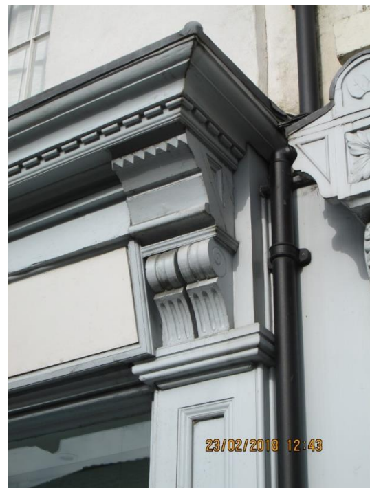
81 Market Street, Ashby. A panelled pilaster carries an unusual bracket; it does not break through the cornice. There is a canted fascia. This shop front has been altered.
