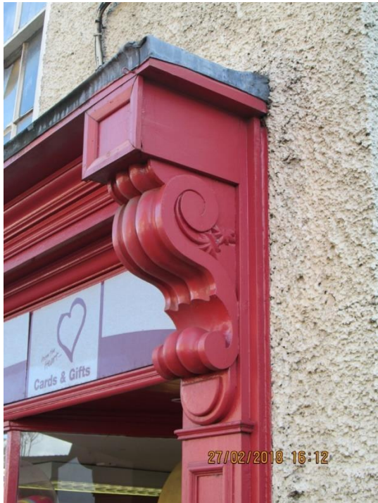
16 Market Street, Ashby. A pilaster with false panelling carries a scroll bracket with a square head. There is a flat fascia with cornice. This shop front has been altered.
