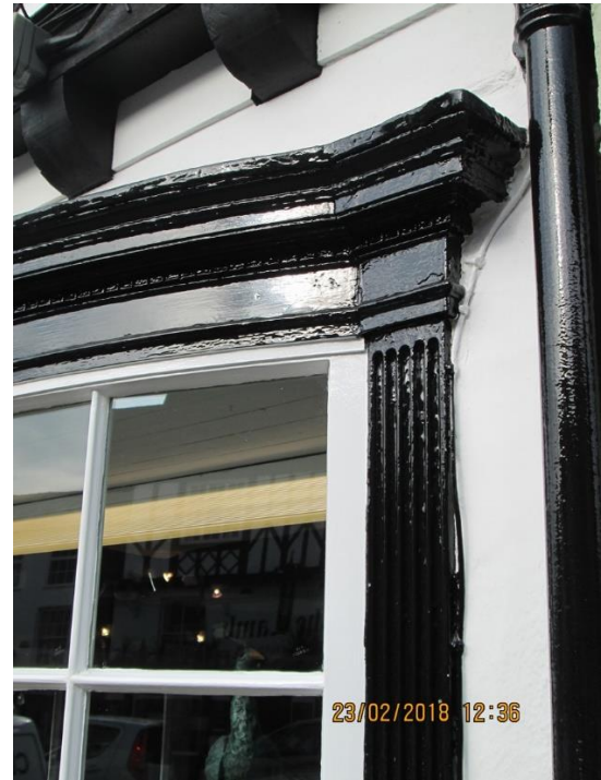
51 Market Street, Ashby. A fluted pilaster with a simple capital supported a shallow frieze and cornice. The shop window is bowed and divided into small panes.
