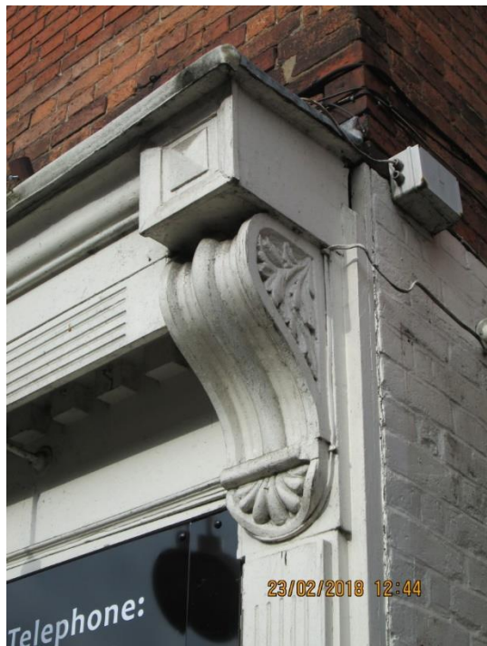
85 Market Street, Ashby. A fluted pilaster carries a scroll bracket with a square head. There is a flat fascia with dentil cornice. The shop display window has been replaced.
