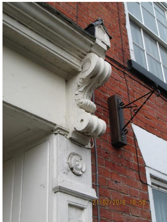
3 High Street, Kegworth. A panellled pilaster with a capital carries a scroll bracket with a gabled head. There is a flat fascia with cornice. Note the panelling in the door recess.
