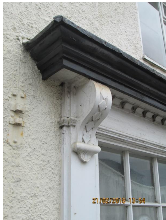
43 High Street, Measham. A plain pilaster carries a scroll bracket; it does not break through the cornice. The shop display window has been replaced. No longer a shop.
