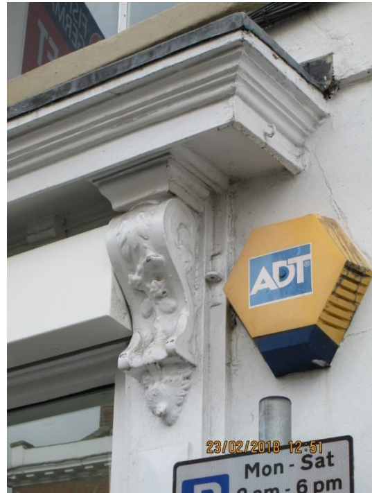
70 Market Street, Ashby. A pilaster with a raised panel carries a scroll bracket; it does not break through the cornice. This shop front has been altered; the fascia is obscured.
