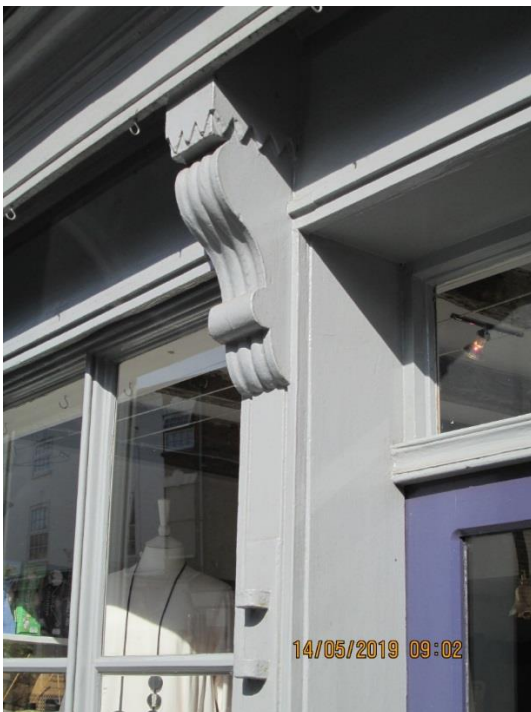
33 Borough Street, Castle Donington. An incised pilaster carries a scroll bracket; it does not break through the cornice. There is a flat fascia. Note the vertical glazing bar.
