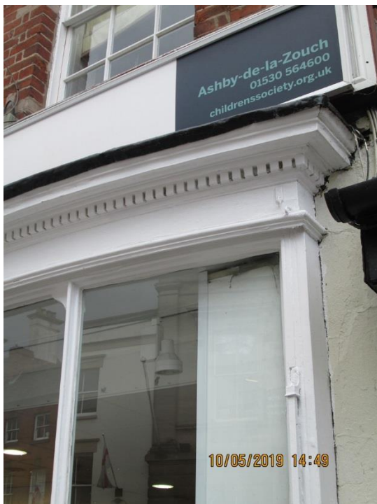
65 Market Street, Ashby. A slim fluted pilaster with no capital carries a frieze and a dentil cornice. The shop window is bowed and contains vertical glazing bars.
