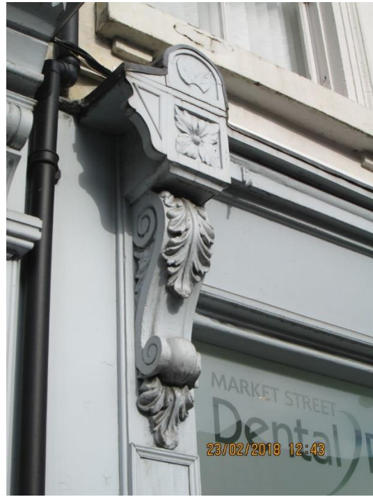
83 Market Street, Ashby. A pilaster with false panelling carries a scroll bracket with a round head. There is a canted fascia. The shop display window has been replaced.
