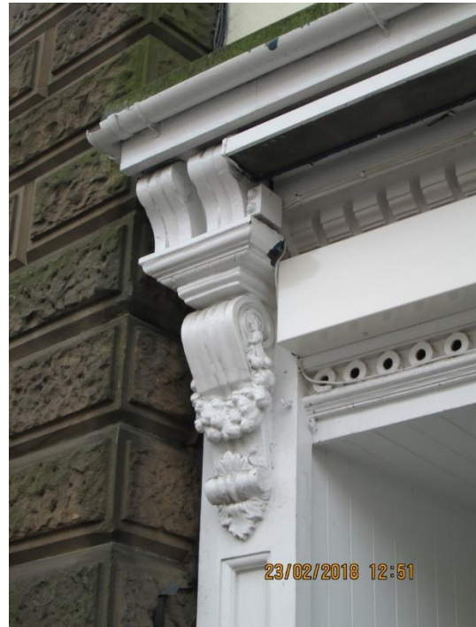
72 Market Street, Ashby. A panelled pilaster carries an unusual bracket; it does not break through the cornice. Altered; the fascia is obscured and the cornice is modern.
