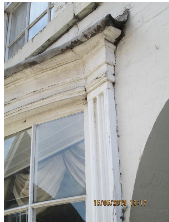
24 Clapgun Street, Castle Donington. A fluted pilaster with a simple capital carries a shallow frieze and cornice. The shop window is bowed and divided into small panes. No longer a shop.
