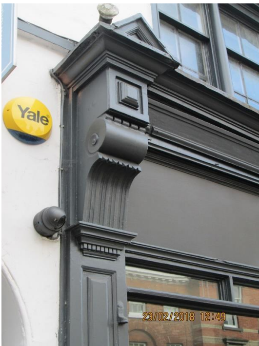
76 Market Street, Ashby. A panelled pilaster carries an unusual bracket with a gabled head. There is a canted fascia. The cornice contains a roller blind.
