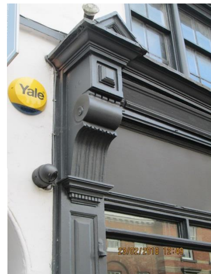
Right: Detail of a typical shop front of the period after c.1850 (76 Market Street, Ashby de la Zouch). A panelled pilaster supports a deep canted fascia and cornice. The fascia is bounded by a bracket. The shop window is flat and contains plate glass; note the narrow overlight.
