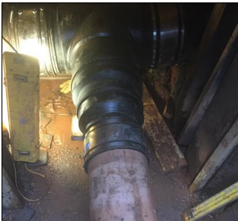
Figure 2: Temporary connection to existing 300m diameter sewer (at the top of the picture) in Station Road.
