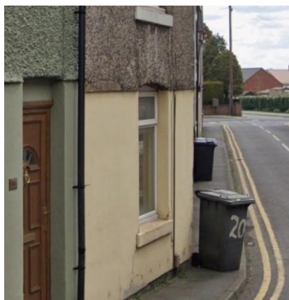
Image 16: Narrow pavement between 14 and 22 Breach Road, Coalville
