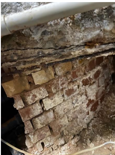
Deterioration Of Supports to Health Suite
