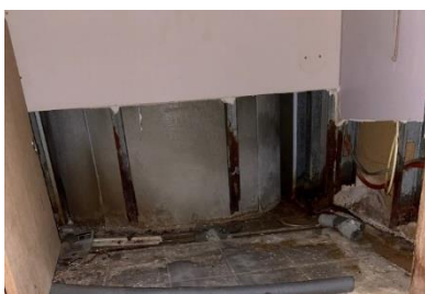
Deterioration Of Supports to Health Suite
