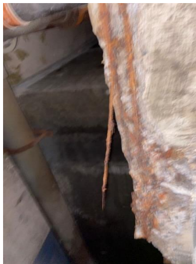
Corrosion of Reinforcement Within Structural Concrete
