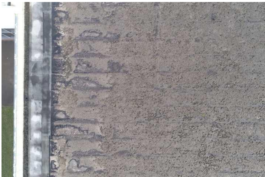
Breakdown of Bitumen Covering
