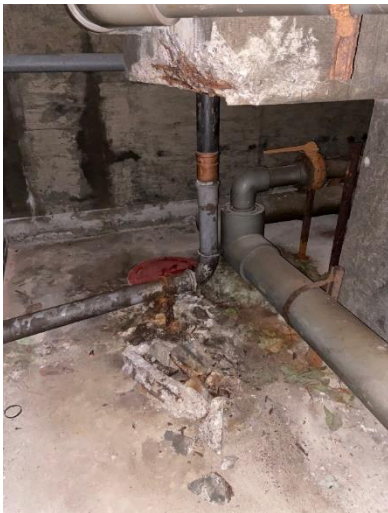
Corrosion of Reinforcement Within Structural Concrete
